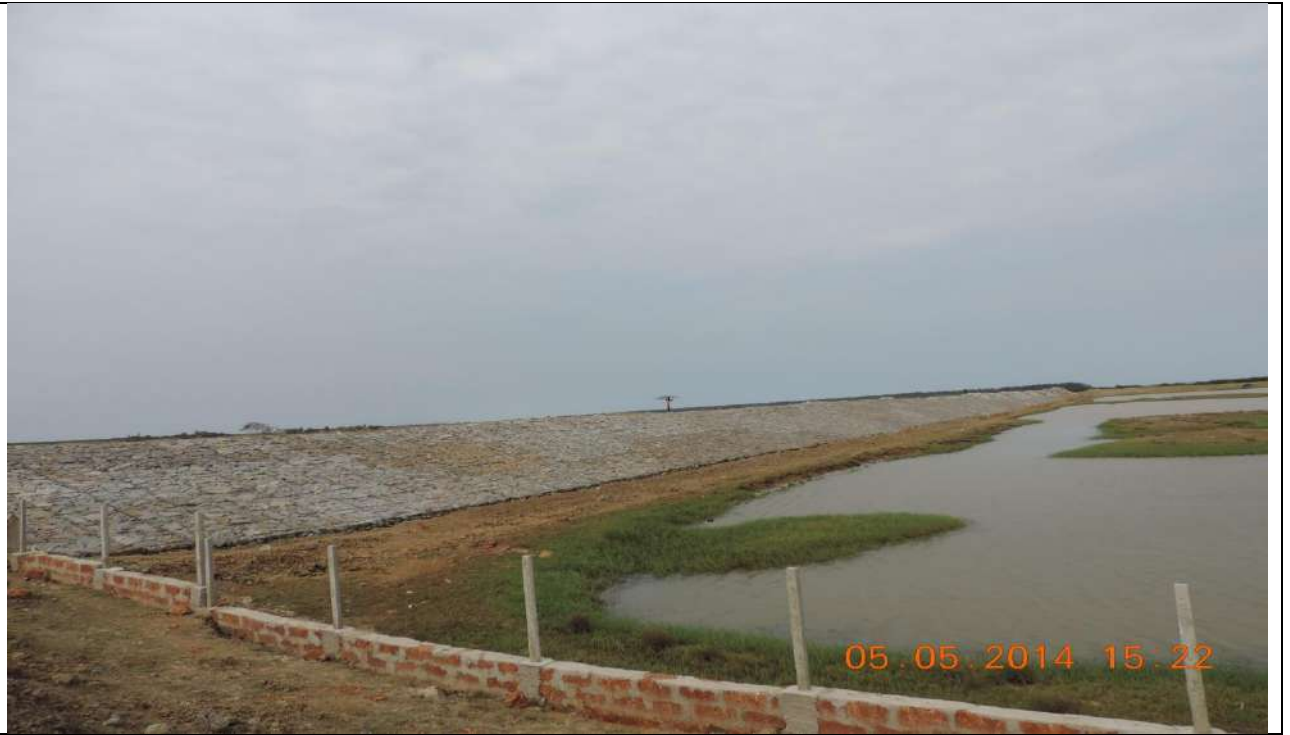
Saline Embankment done through in Jagatsingpur district under NCRMP (2013-16)
