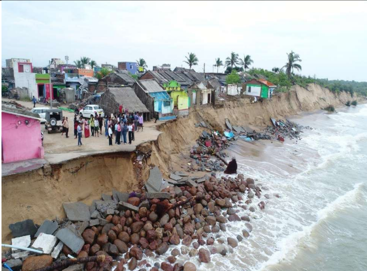
RAMAYAPATANA - Shoreline erosion during cyclone "Titili " on 11.10.2018
