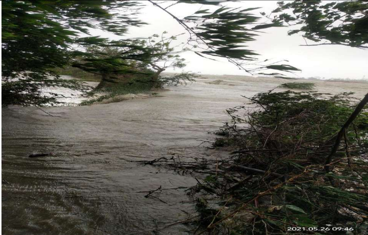
Parikhi Saline embankment submerged due to storm surge of cyclone "YAAS"
