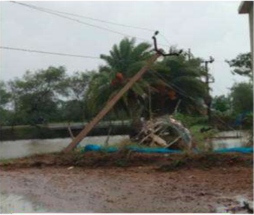
Conductor Snapping
