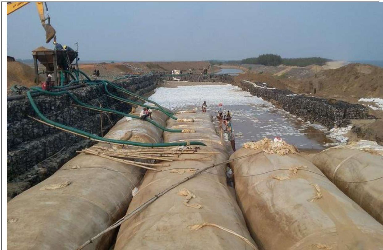
Laying of Geo Tube during construction at Pentha in Kendrapada district
