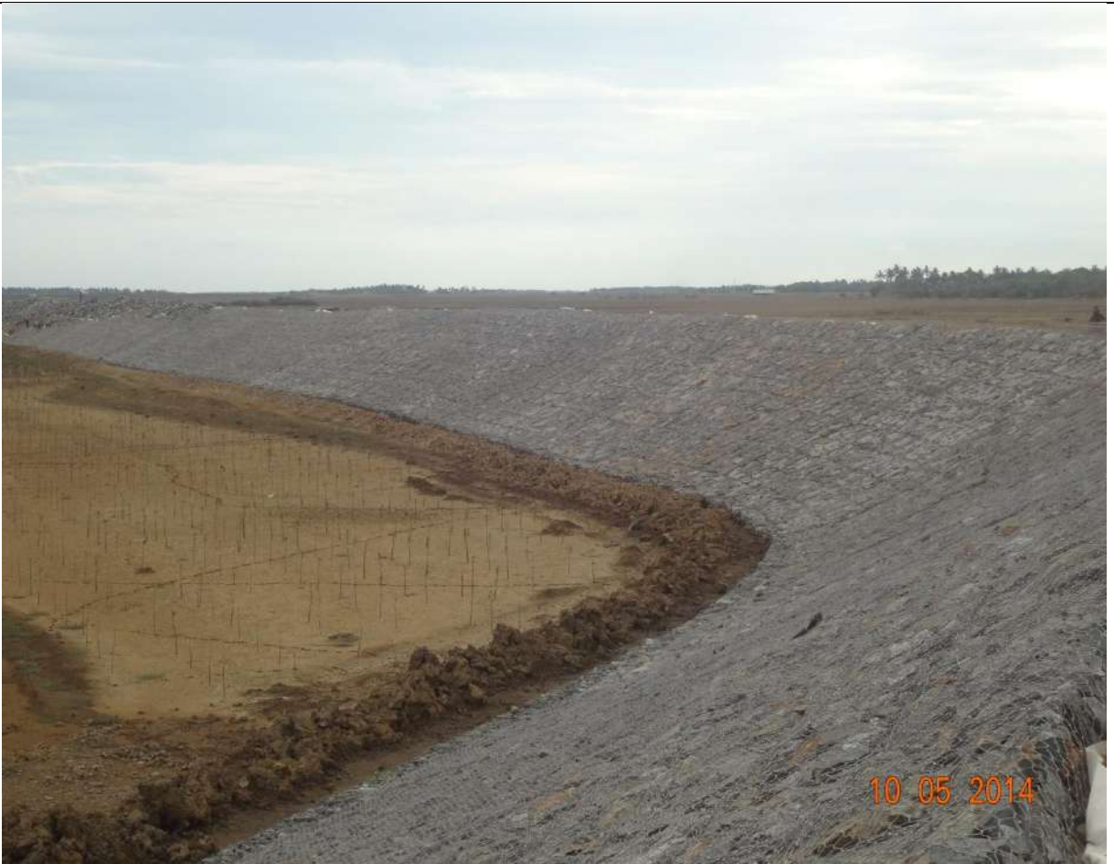
Saline Embankment done through in Puri district under NCRMP (2013-16)
